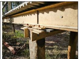
Defect 2 - Missing Nut
