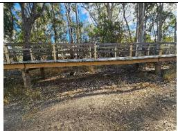
Defect - Sagging beam span 4
