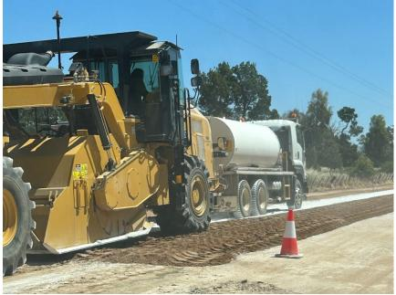
Bunnaloo Road construction, pad foot rollers compacting and pavement mixing.
