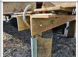
Defect 3 - Anchor bolt not installed
