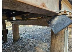
Defect 5 - Elastomeric bearing moved
