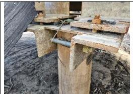
Defect 1 - Bolt not through timber
